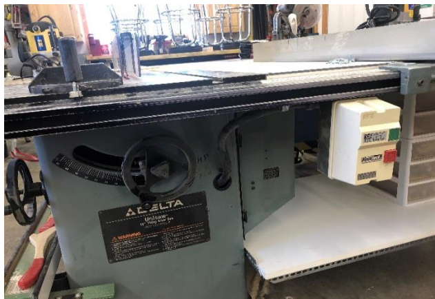
(Another wiring priority is to move the main switch on the Unisaw to the left side of the blade.)
